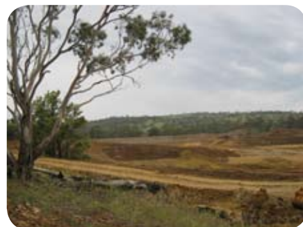
The dam site nearing completion.
